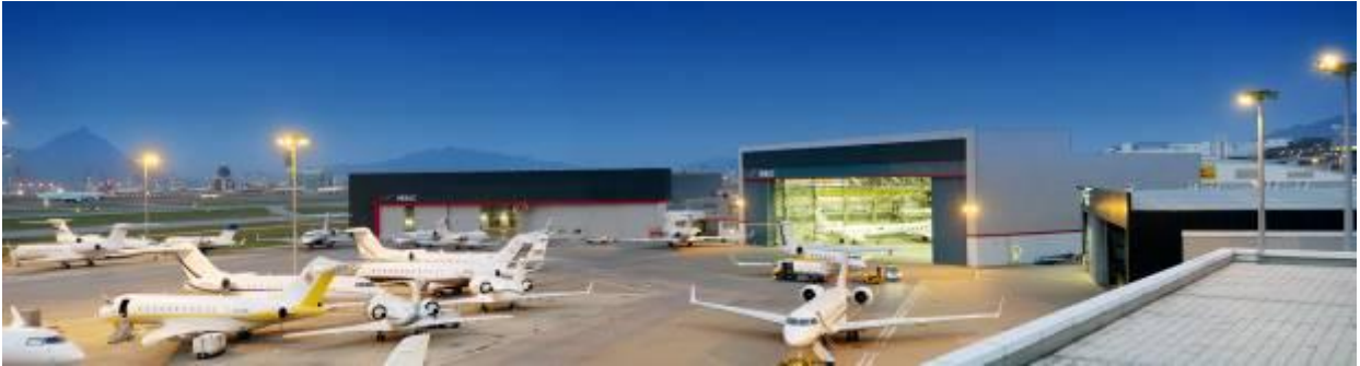
(From left to right) Hangar 3, hangar 2 and hangar 1
